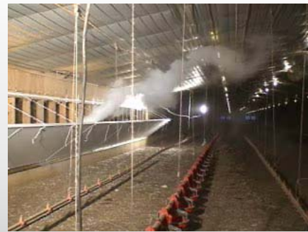
Tunnel door air flow pattern
