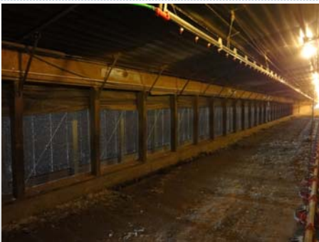
Tunnel curtains have to be closed significantly to have a similar effect
